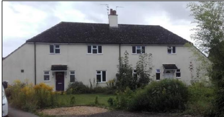
East side of Uffington Road: social housing built in the 1920s
